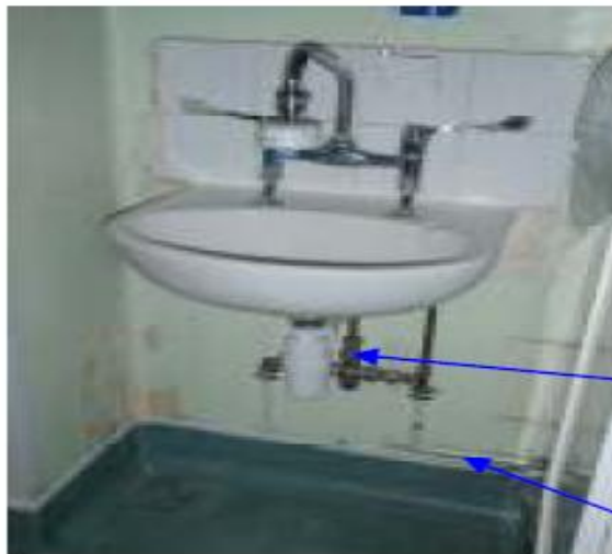
Figure 9: QE/2/1 ITU Bay 1; The cold water pipe is probably holding stagnant water
