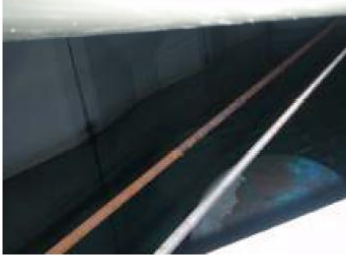
Figure 1: Inside the main cold water storage tank; (001152) = 20.3°C.
